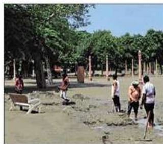
Staffers are cleaning the surface-level silt, removing unwanted plants and repairing infrastructure
